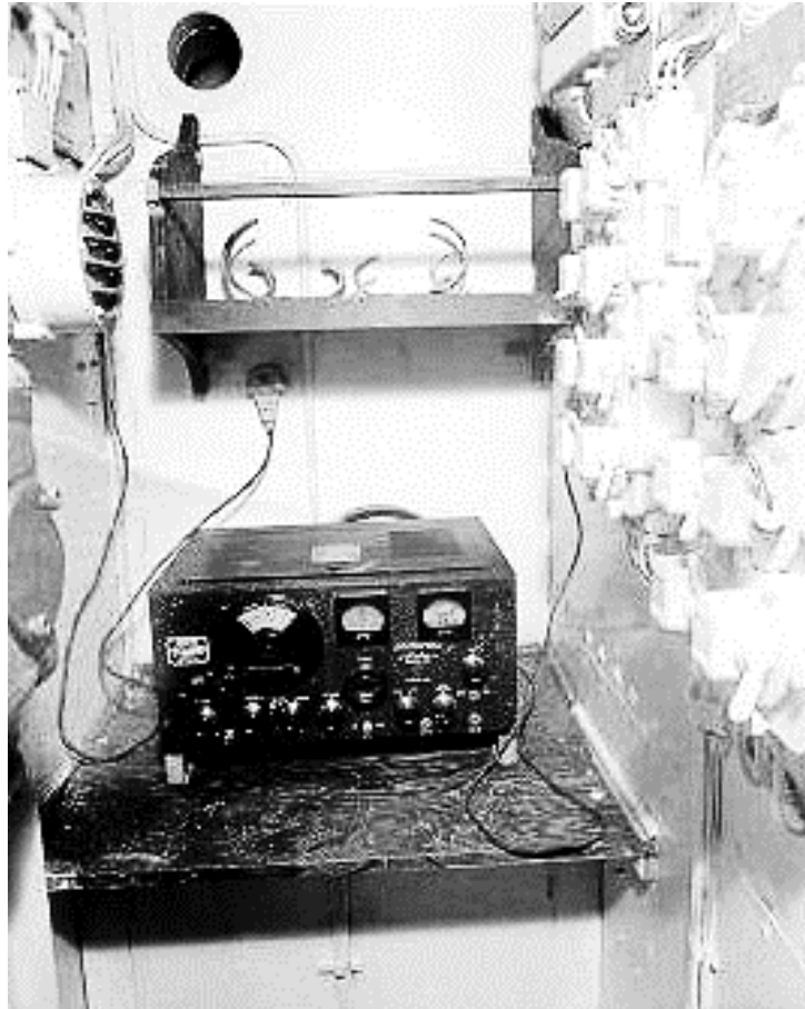
This is the actual Headache Office aboard HMCS HAIDA during WWII. Pictured is the Hallicrafters S-27 receiver which was removed in 1949. (RCN photo HS 1749-59 taken in 1946).
