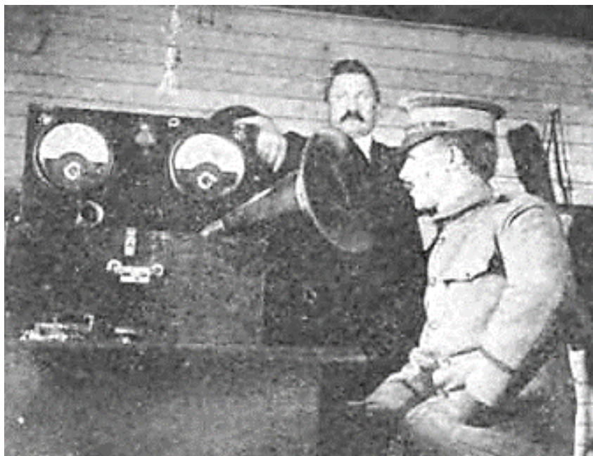
Transmitting an order by wireless phone. Wooden box contains entire apparatus, making it easily available for military field work.
