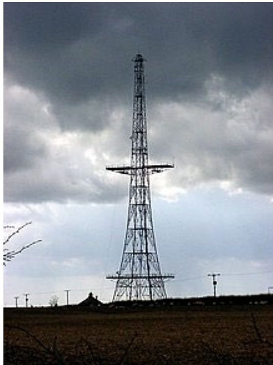
A Chain Home transmitter antenna, part of one of the first comprehensive radar systems.
